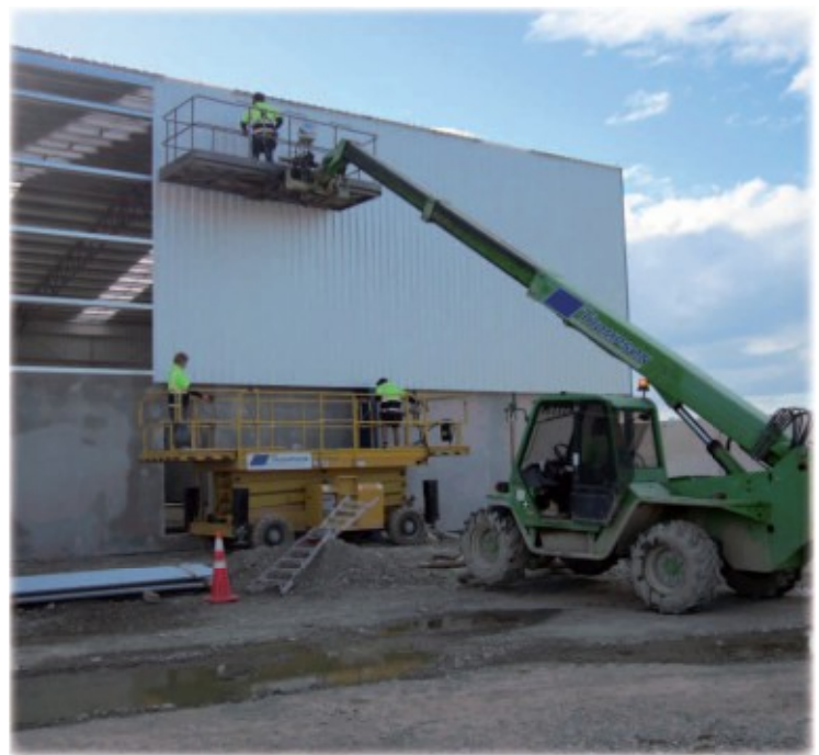
East wall cladding being installed
