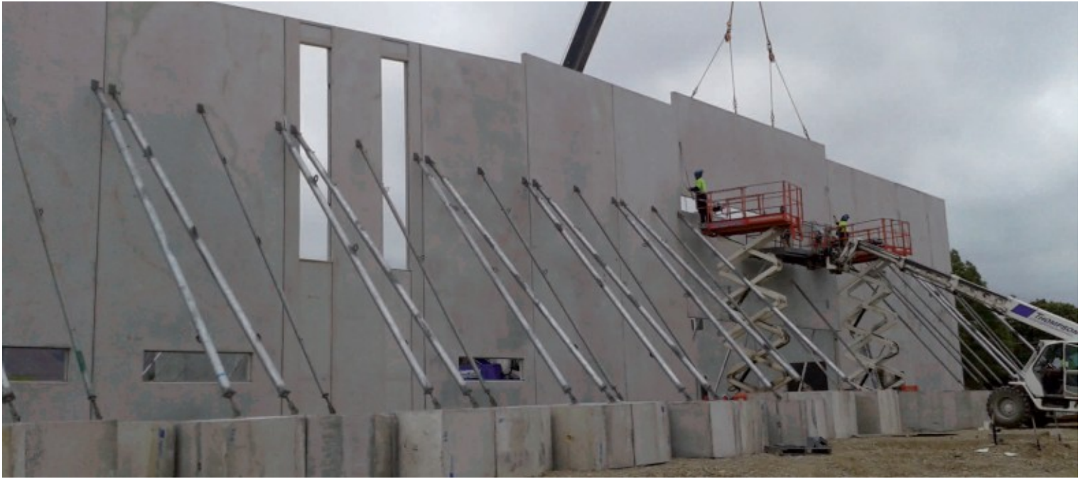
Panels being installed
