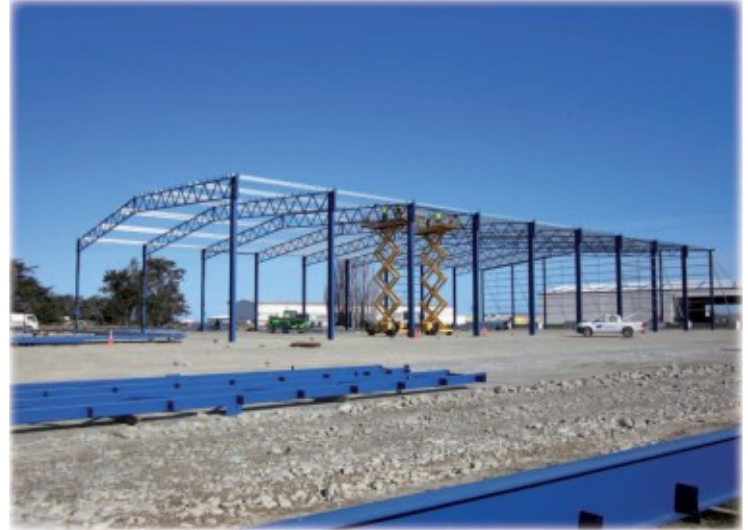
Half of the trusses erected
