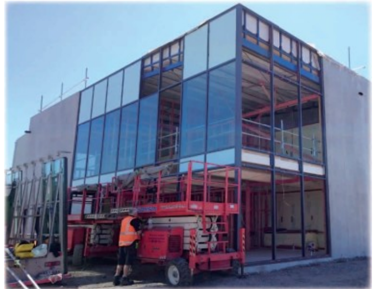
Glass being installed
