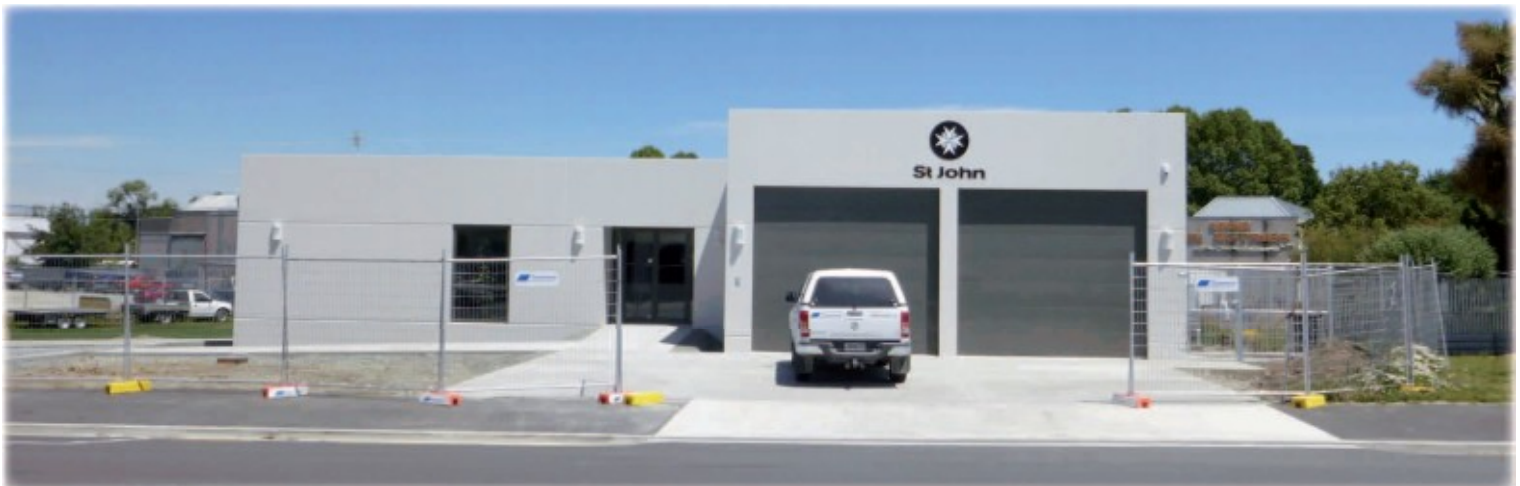
Nearing completion December 2015
