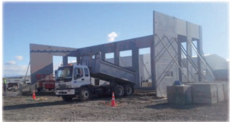
First office panels installed
