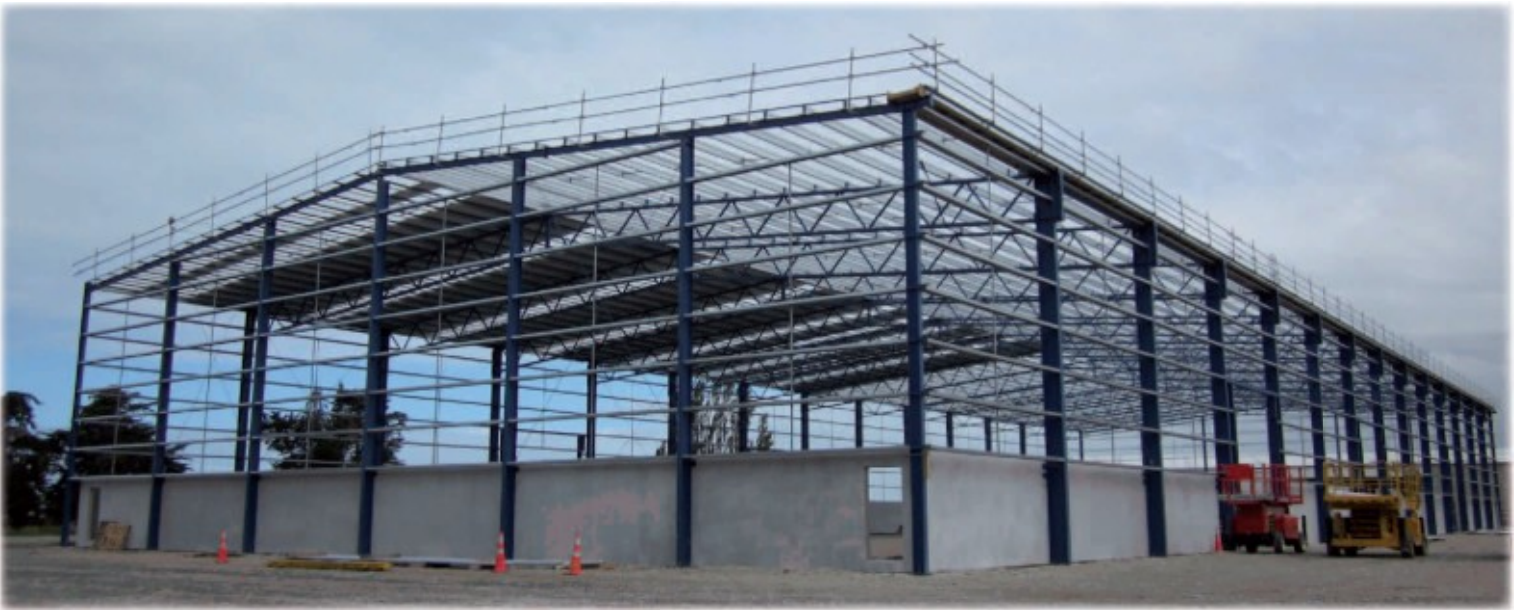
Panels installed and roof cladding beginning
