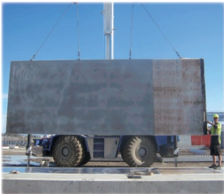
Panel being lifted from the bed with protection cover
