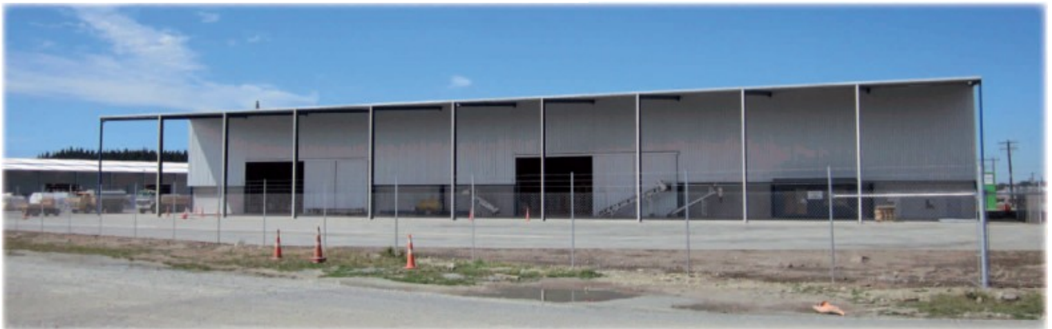
Zealyn Bulkstore completed, Washdyke
