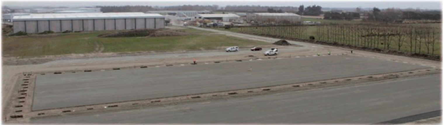
Pads for steelwork in construction
