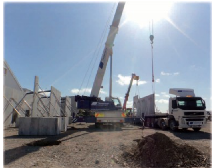
Panels being transported to site and installed
