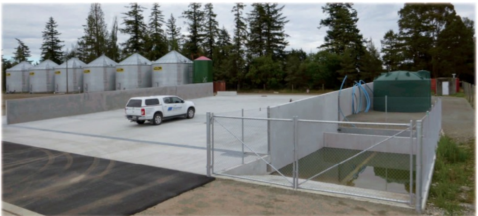
Truck wash completed
