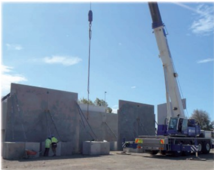
First panels being installed
