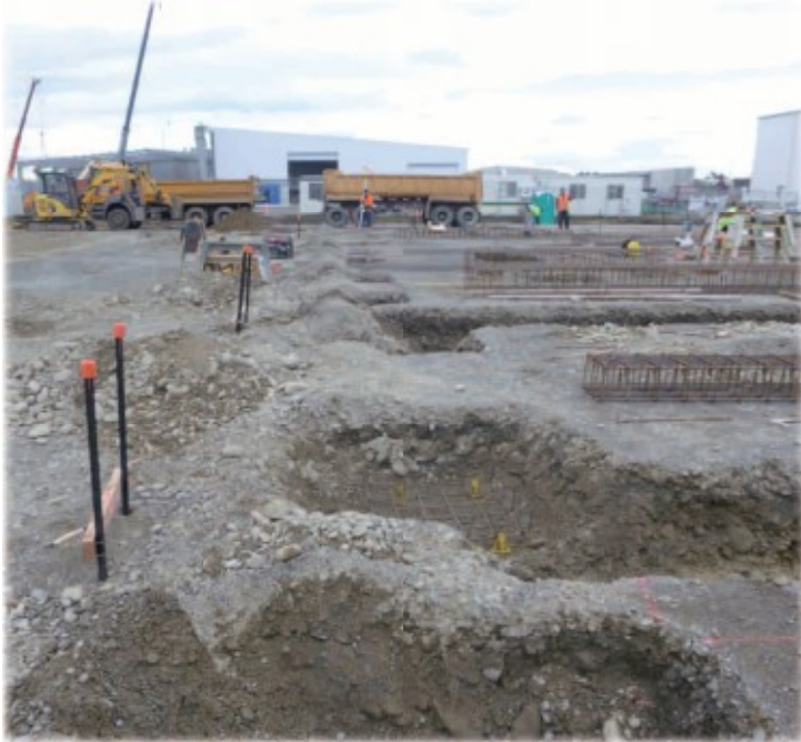
Foundation works in progress
