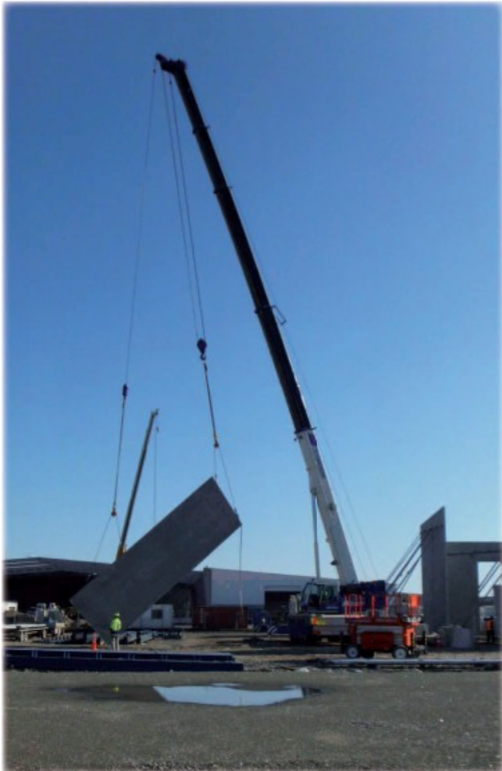
Panels being installed for the office
