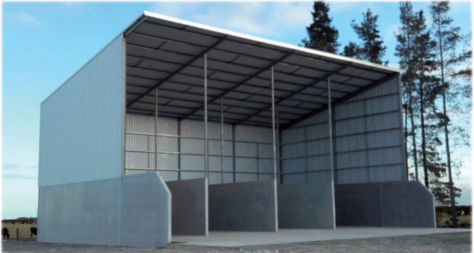
Fertiliser bulkstore completed
