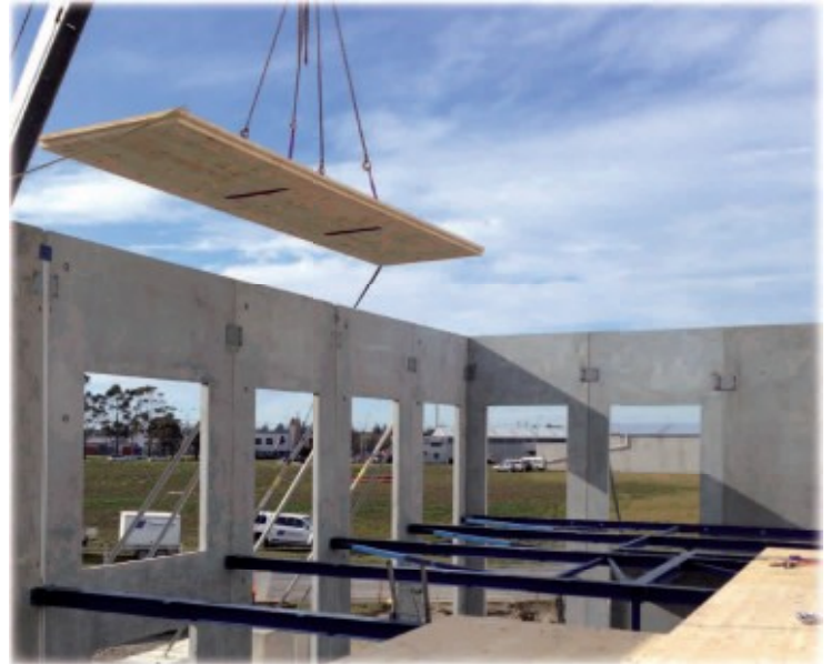
Cross laminated timber flooring being installed
