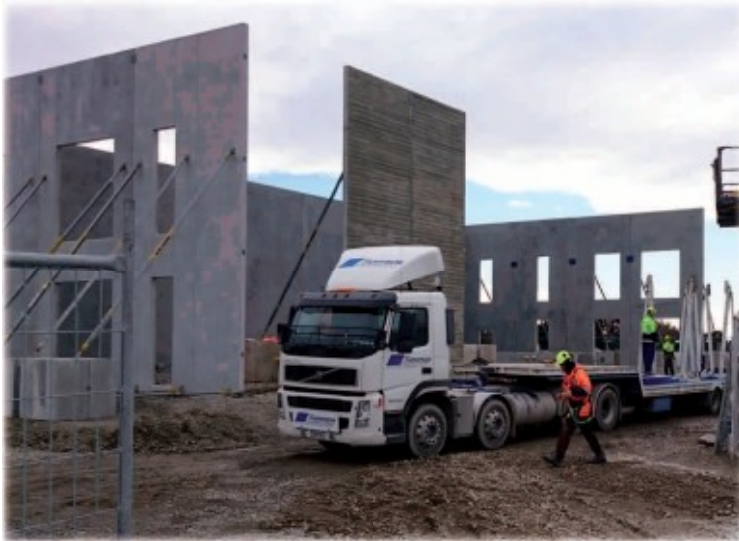
Office panels being installed
