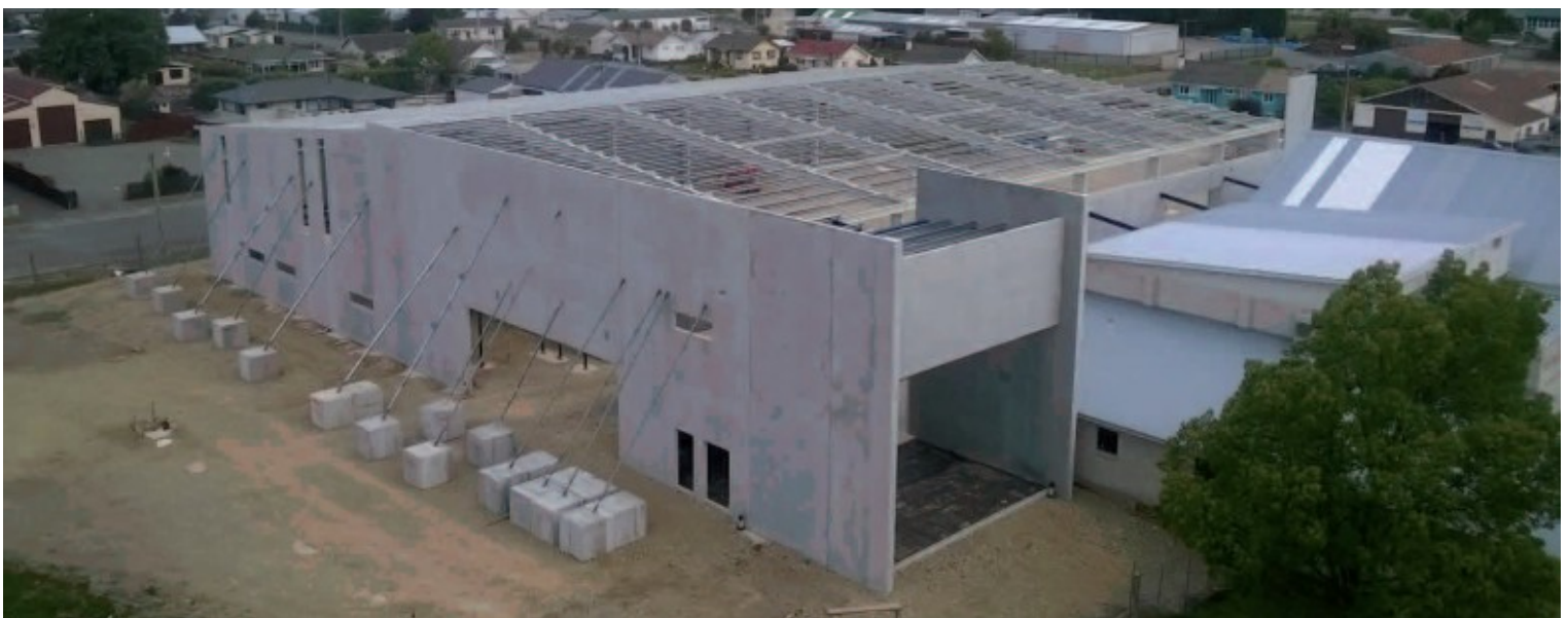
Waimate Stadium in construction
