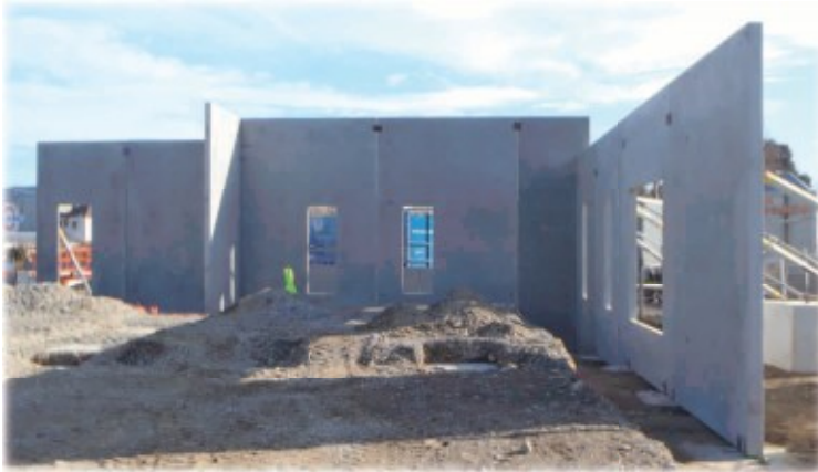
First panels installed
