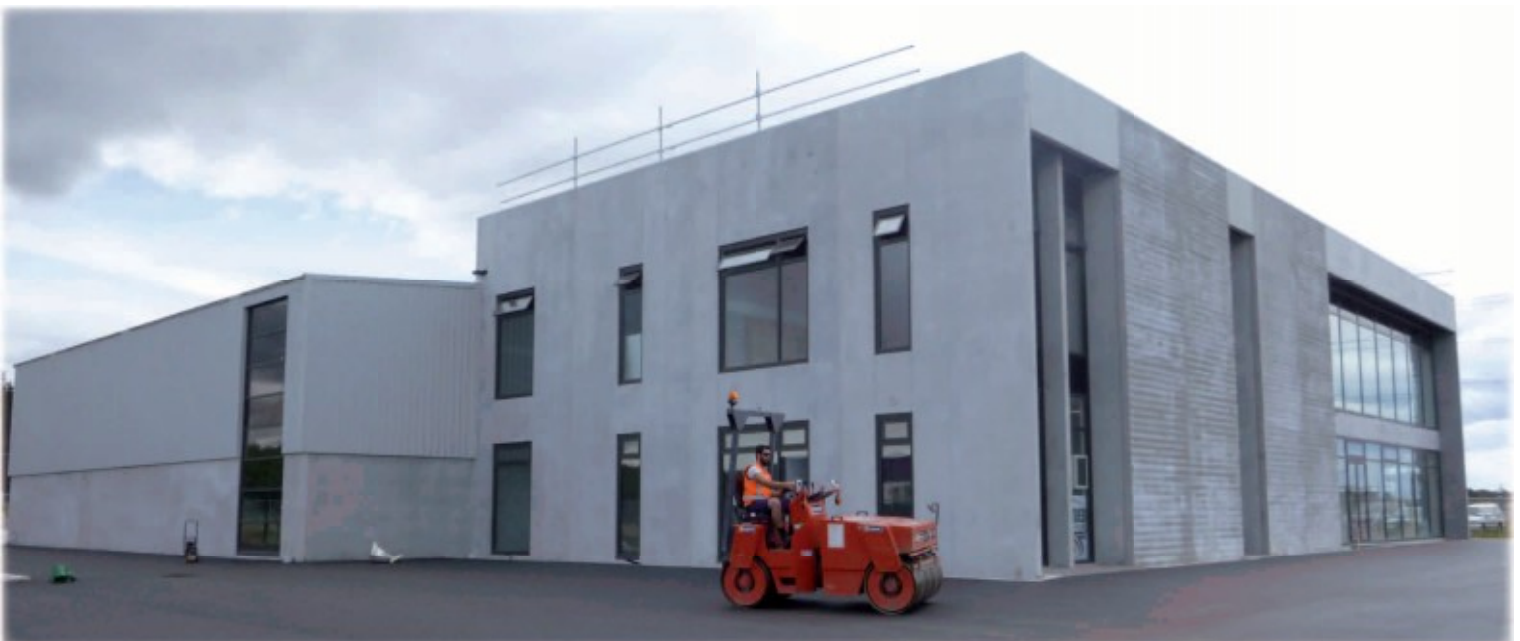
Office, cafe and warehouse in construction with asphalt laid December 2015
