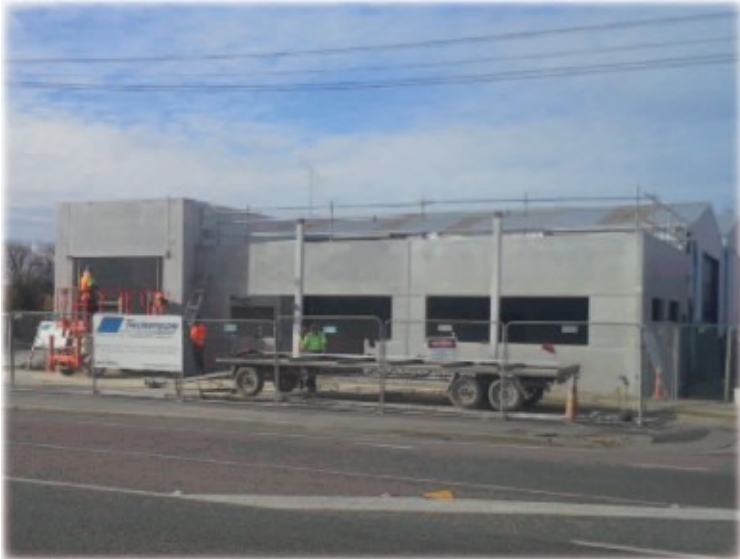
In construction with all panels installed
