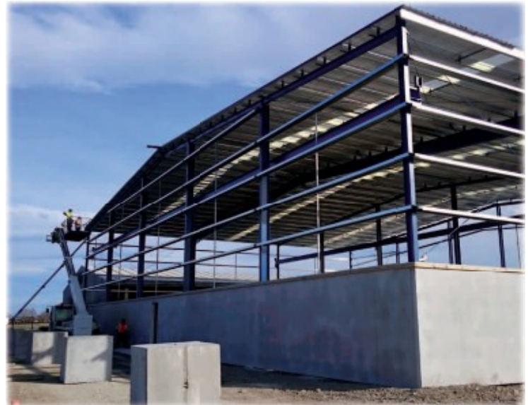
Roof being installed
