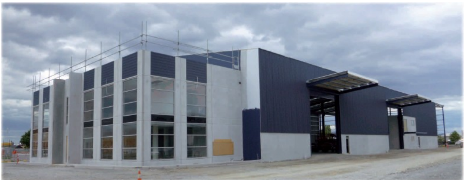
In construction Dec 2015
