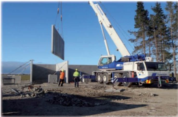
Precast panels being installed
