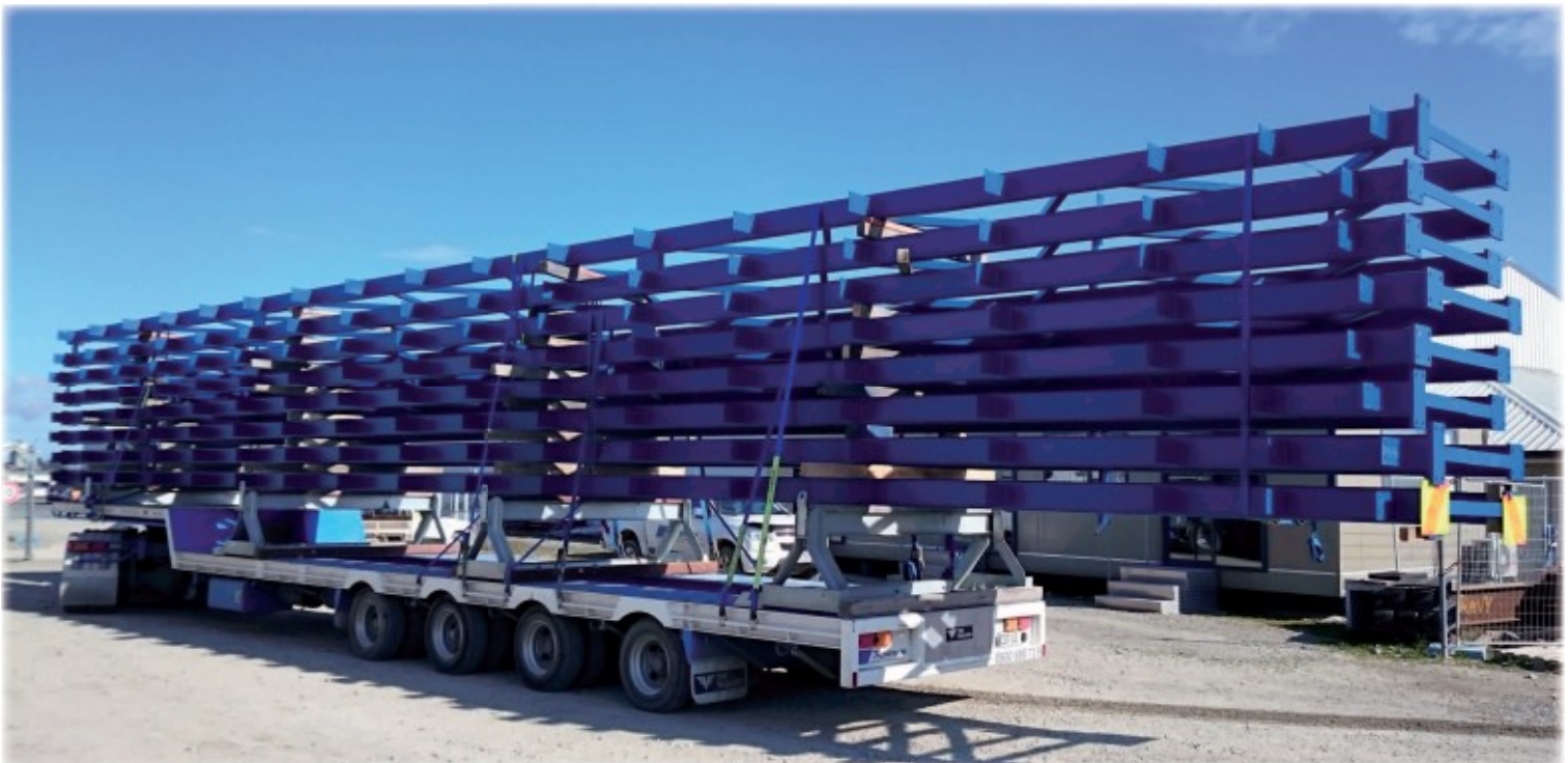
Steelwork being transported to site by Thompson
