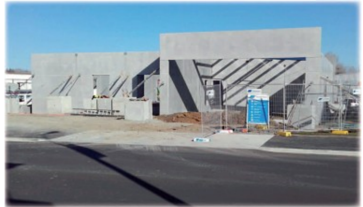
Panels installed for the ambulance bay and entrance
