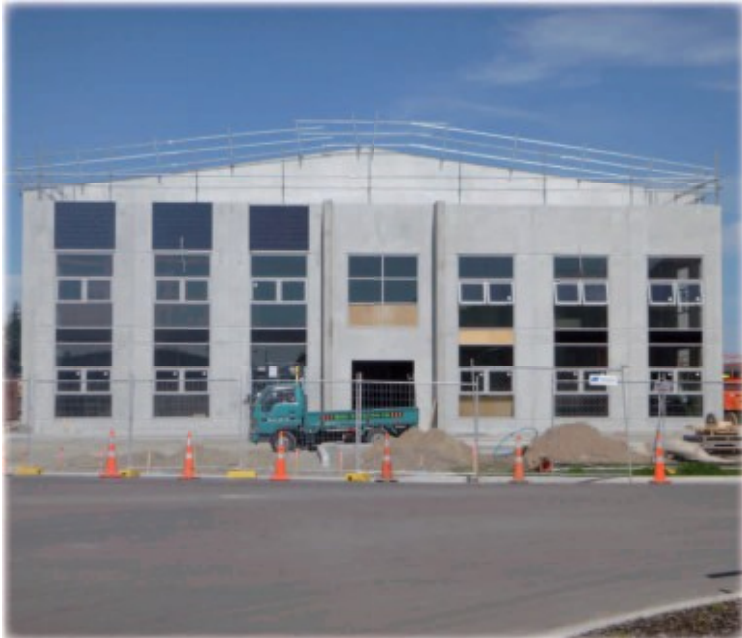
Two storied office in construction with painting beginning
