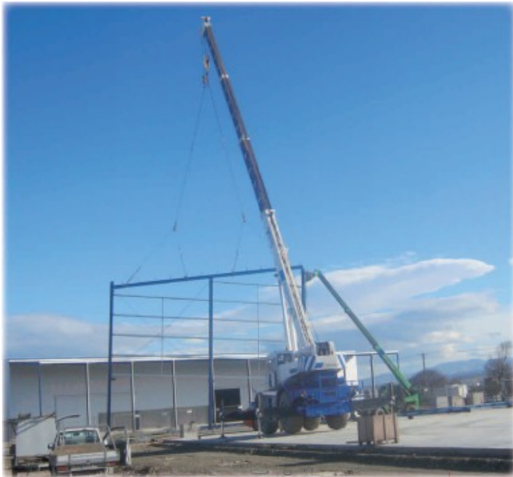
First truss being erected
