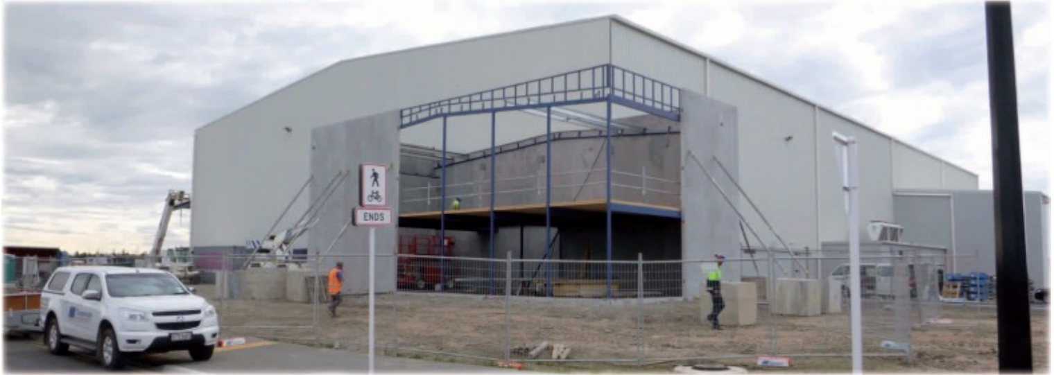
Steelwork, precast panels and metra panel second storied floor installed
