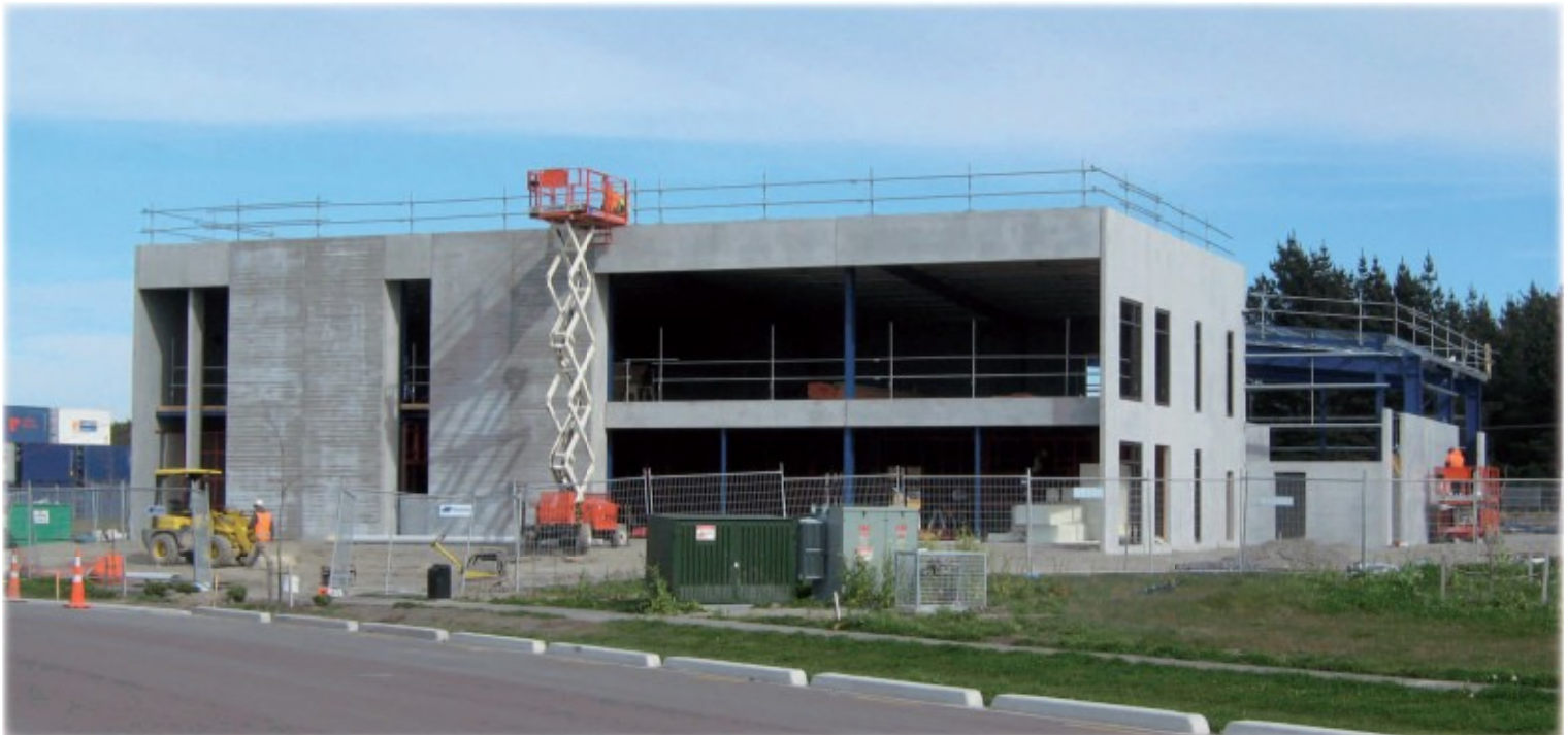
Office panels, warehouse panels and steelwork installed
