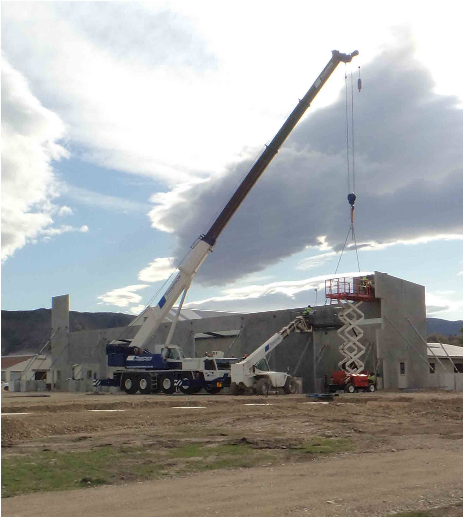
Waimate Event Centre Stage One panels being installed
