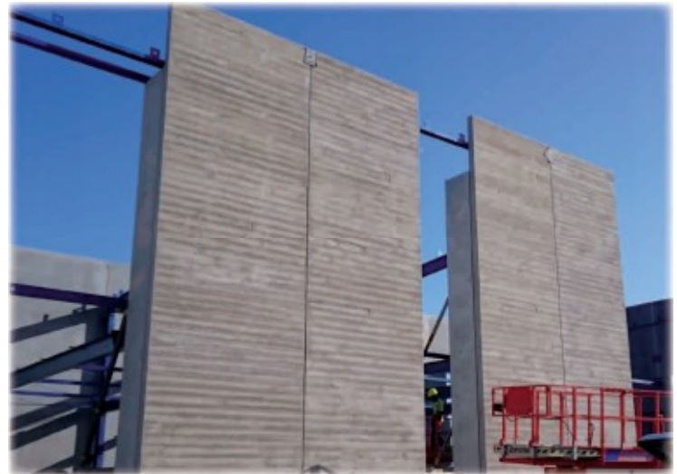
Architectural textured panels installed
