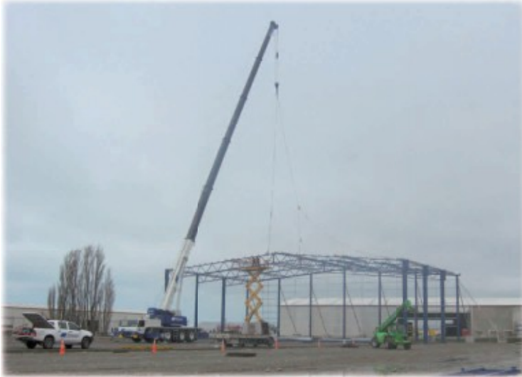
80T crane erecting the steelwork
