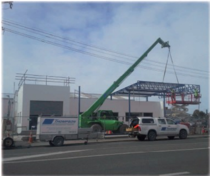
Forecourt canopy being installed
