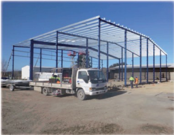
Steelwork erected and purlins installed
