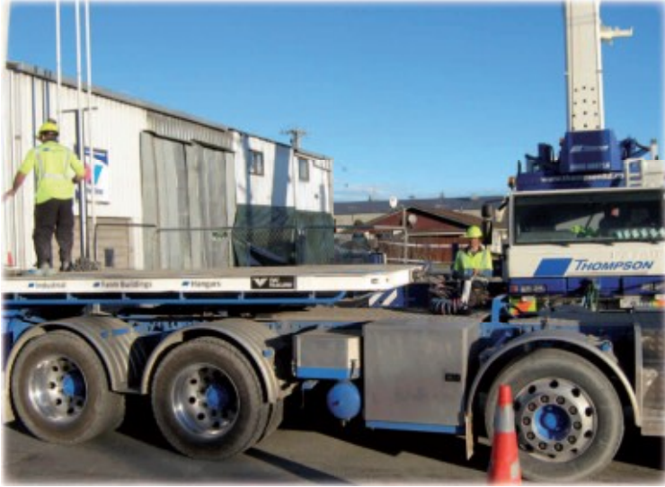
Getting geared up to start installing panels
