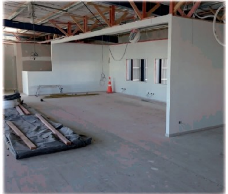
Fit out of offices in progress
