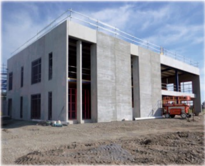
In construction September 2015
