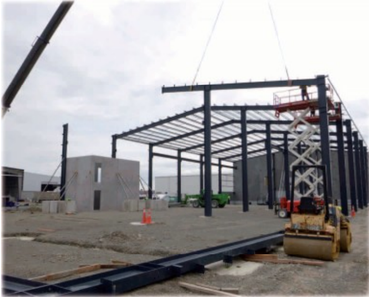
Warehouse steelwork being erected
