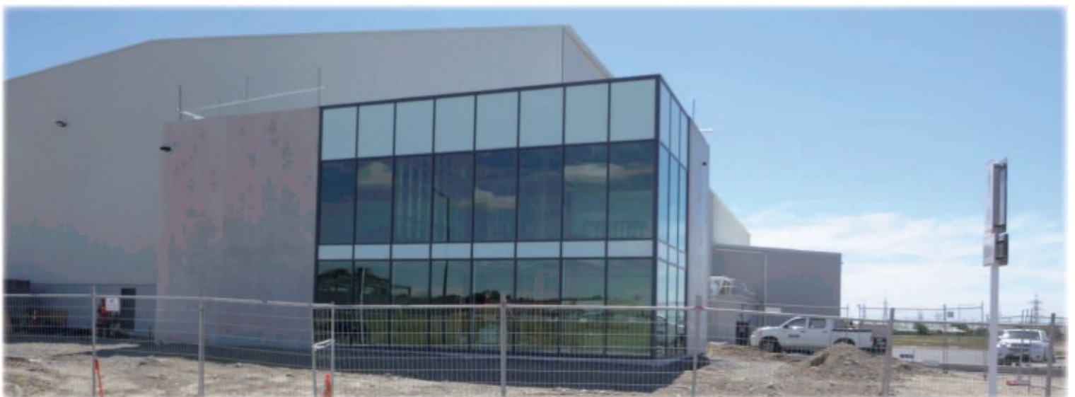
In construction December 2015
