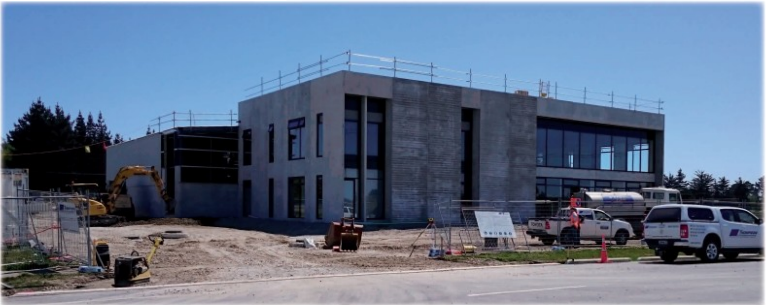
Warehouse and offices in construction
