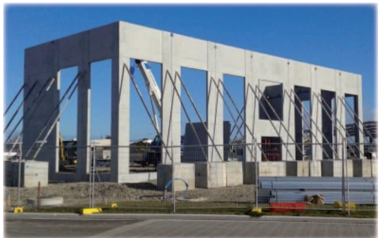
Office in construction
