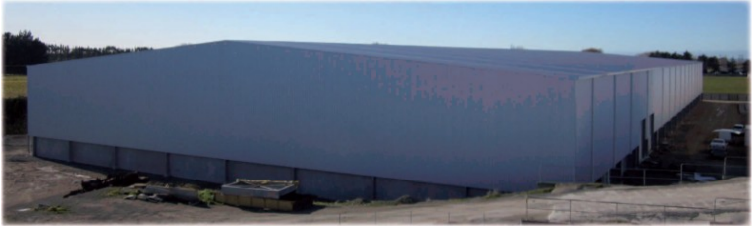
Rooney Earthmoving (Shed 11) 67m clear span bulkstore completed, Washdyke
